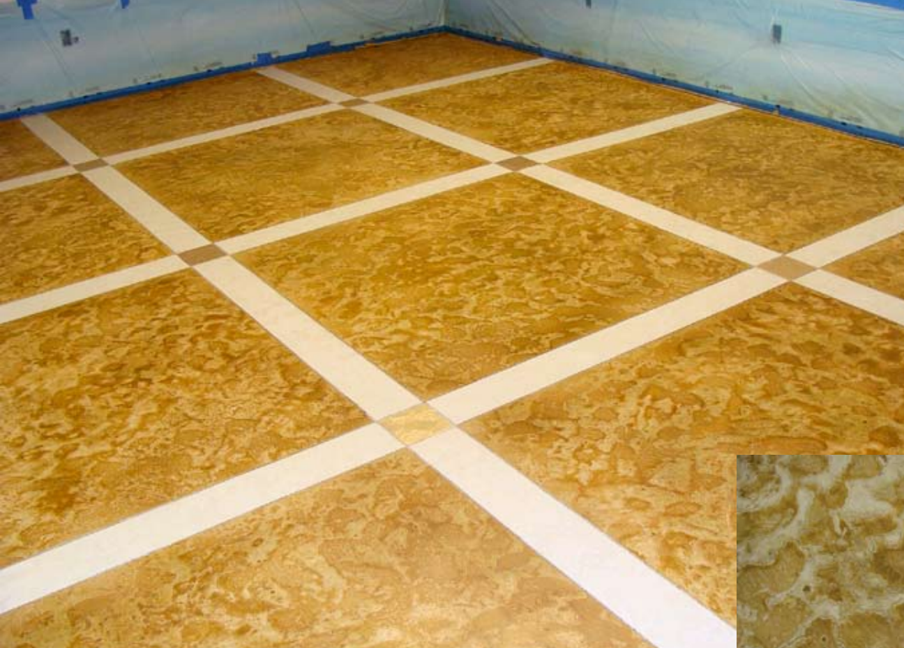
A skip-troweled microtopping with Miracote's architectural water-based stain, Mirastain II. There are two colors used on this floor. One is a liquid pigment (ColorPax-LIP Tiger Gold) and the other is a dry metallic pigment (Pale Gold).
