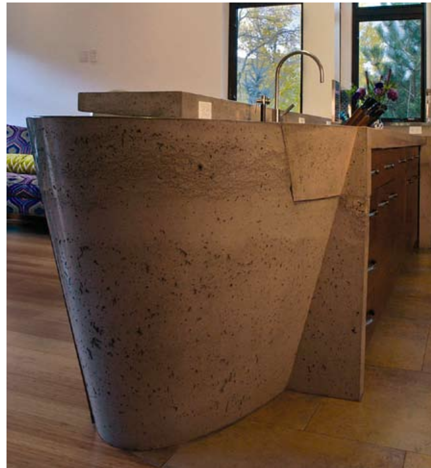
Bug holes, defined horizontal laitance and color variegation create visual interest in this cast-in-place vertical, by artisan Sean Dunston, with Concrete Jungle, of Colorado Springs, Colo.
