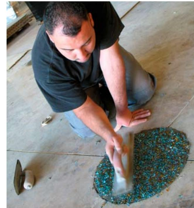
Jellybean Glass from American Specialty Glass is floated into concrete to represent pier pilings. Different colors of tumbled glass were also scattered into the concrete throughout the store to suggest sand on a beach.
