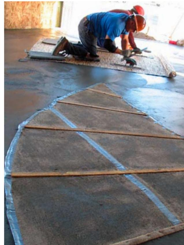
Sail stamps were made out of burlap, duct tape, bamboo and redwood battens. After a test run, they were completed with a combination of applied and impressed finishes and colors.
