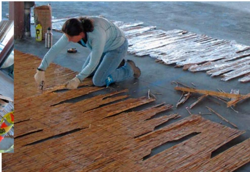
Bamboo fencing was cut into cloud graphics and rolled on top of the hard, yet still green concrete. The sheets sat on top of the concrete for ten days and weighed down in various spots to promote differential curing.
