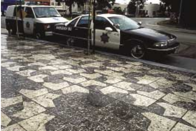
"Sheriff's Star Plaza and Lobby" is a collaboration between Seattle artist Vicki Scuri and San Francisco fabricator Buddy Rhodes. Constructed with monolithic black and white precast concrete pavers, black area "voids" were in-filled with white, and vice versa
