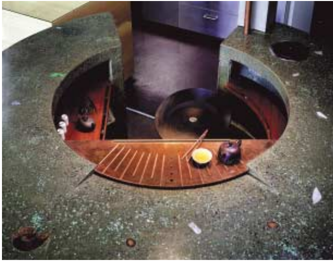
This countertop, by Fu-Tung Cheng and Cheng Design, is a blend of old school discipline and new school intimacy. There is as much attention to the details and to the finish of the tea bar as to its form. Note the simulated ammonite fossil and other integral embeds
