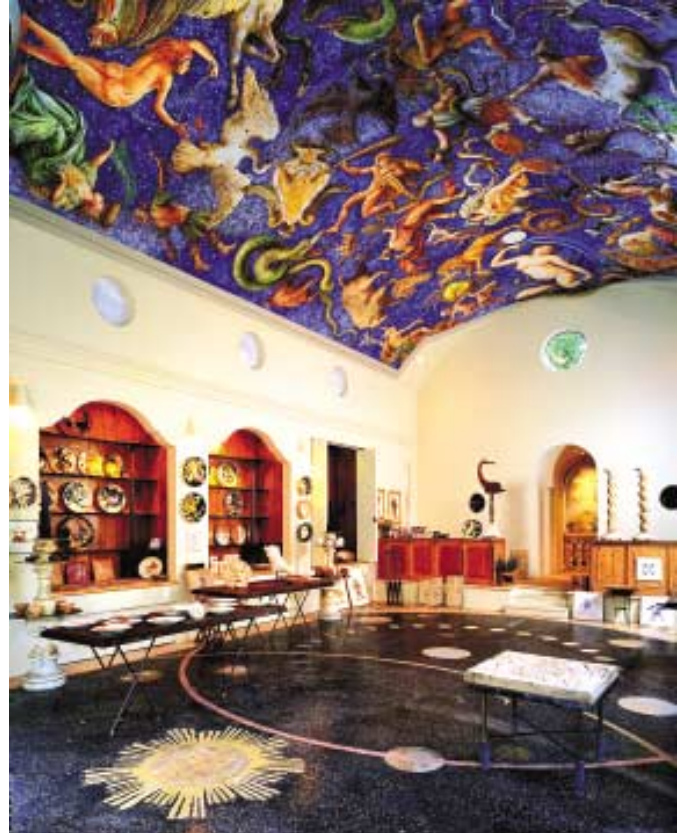
Floor of Ca'Toga, Galleria d' Arte by Venetian artist Carlo Marchiori, combining old school concrete and terrazzo techniques with out-of-the-box, hand-packed precast planetary elements
